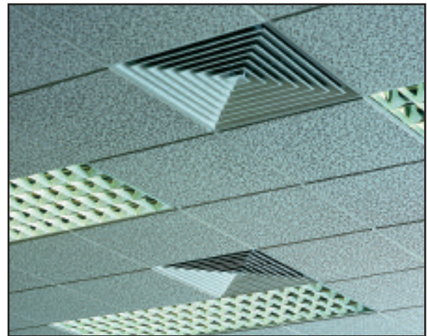
Louvre face diffusers in a typical installation
