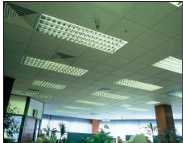
Louvre face diffusers in a typical installation
